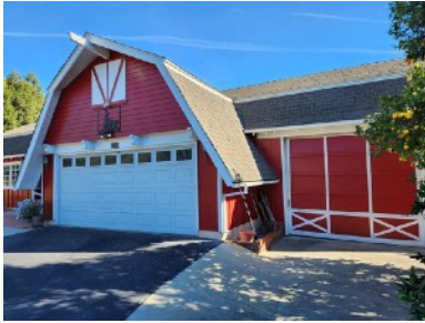
The Bird residence. Thomas built the addition on the right.
